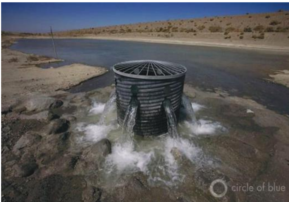
Figure-17a A groundwater recharge facility for the Coachella Valley adds water imported from the Colorado River to the valley's main aquifer and prevents the land from sinking and damaging the surrounding infrastructure.
