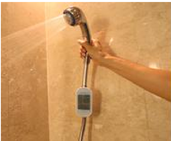
Figure-24: A smart meter is installed on the showerhead to track water usage
